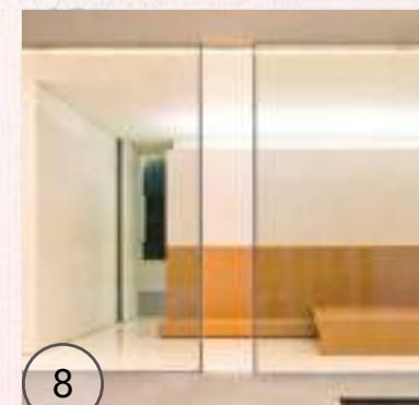
8 LOW IRON GLASS WITH BLACK ALUMINIUM MINIMAL FRAME
